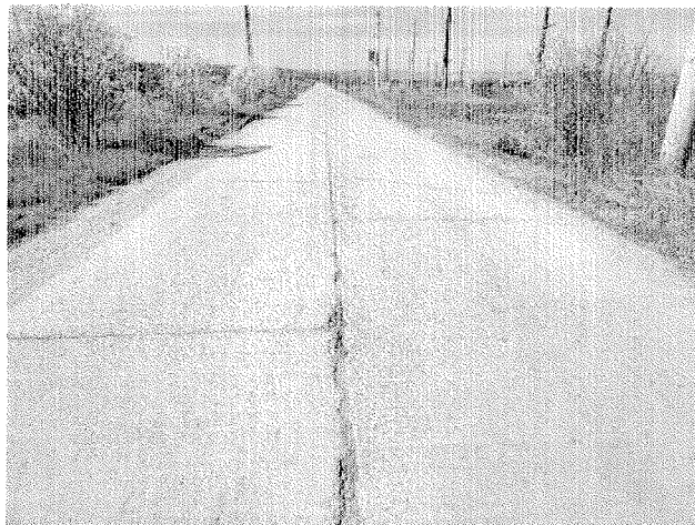
Rosturi deschise colmatate, rupturi de colt
